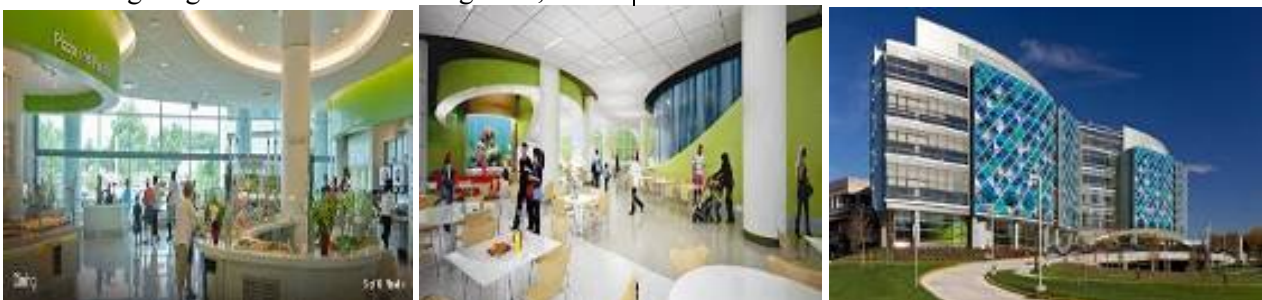
Figure 27:the diagonal pattern and the triangular colors suggest that the glass is modular in that way, they're really rectangular sections of glass that have been twisted with battens on the outside of the building to create the diamond grid.
