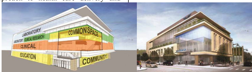
Figure 10 : Exterior of Winthrop University Hospital Research and Academic Center. Courtesy of Perkins
